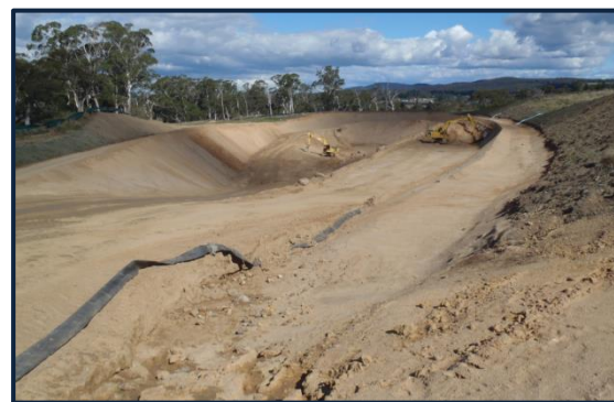
Rehabilitation and construction and assessment.
